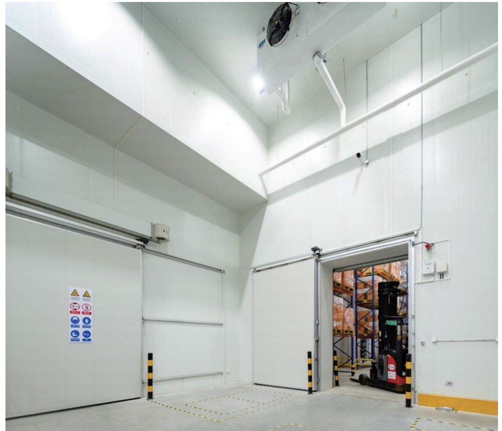
● QICHENG SUPPLY CHAIN BEIJING SHUNYI PROJECT
